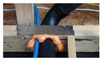
**Correction Notice:** The required strapping was missing at the gas main top plate location. Notches or bored holes were observed at the top plate which were 50 percent or greater of the top plate width without the required 1 1/2" galvinized metal tie fastener with 6-16d nails at each side of the notch or hole. We recommend installation as required. **(R602.6.1)**
