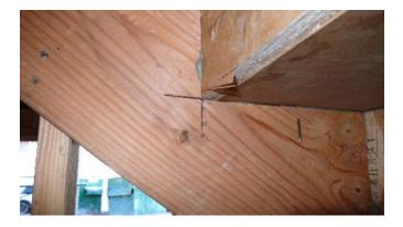
13. **Correction Notice:** The thrust blocking at the bottom of the staircase was not secured to the floor with J-Bolts. A minimum 2x4 thrust block must be secured to the floor and notched into the carriages to prevent slippage. We recommend installing the properly secured and notched thrust blocking as required.
