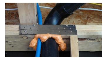
4. **Correction Notice:** The required strapping was missing at the gas main top plate location. Notches or bored holes were observed at the top plate which were 50 percent or greater of the top plate width without the required 1 1/2" galvinized metal tie fastener with 6-16d nails at each side of the notch or hole. We recommend installation as required. **(R602.6.1)**
