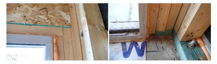
3. **Correction Notice:** The top plate straps were missing the required nailing at the left side DWV piping area. Notches or bored holes were observed at the top plate which were 50 percent or greater of the top plate width without the required 1 1/2" galvinized metal tie fastener with 6-16d nails at each side of the notch or hole. **(R602.6.1)**
