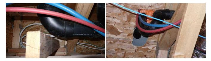
21. Correction Notice: The drain line at stair area was observed to have a negative slope. Drainage fittings should be designed to maintain a one fourth unit verticle in 12 units horizontal (2 percent slope) grade. We recommend that the pipe installation slope as required. **(P3002.3.1)**
