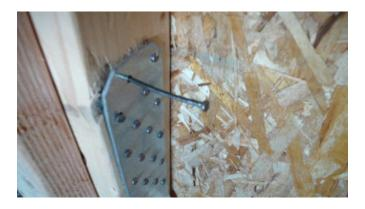
6. **Correction Notice:** Continuous utility straps were observed in several locations with incorrect fastener sizes. 1 1/2" .131 nails were observed, Simpson listed straps have a minimum of 10d .148 nailing unless a load reduction of 30% is specified in the approved plans and specifications. We recommend that the CS18 strapping be installed with the recommended fasteners unless otherwise noted in the plans. (Approved Plans & Specifications) (Manufacturers Installation Instructions)
