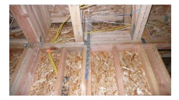
7. **Correction Notice:** The garage shear wall sheathing was not nailed to the doubled studs of the hold downs as required. We recommend that the required nailing be installed for the design performance rated by the manufacturer. **(Manufacturer's Installation Instructions)**
